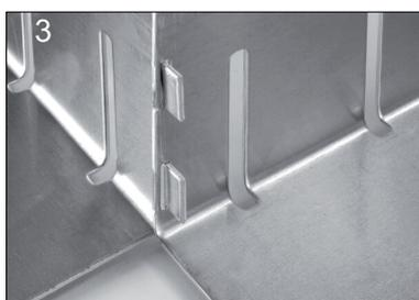
3 Inserting the joints
